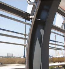
All BLÜCHER® EuroPipe rainwater downpipes are vandal-resistant, combining the aesthetically pleasing look of stainless steel with vandal-proofing of the downpiping and the other inherent benefits of stainless steel material.
